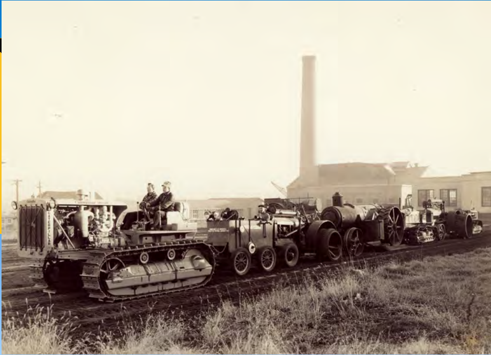
This pre-1936 photograph of the test track located on East Campus, shows the campus steam plant in the background. The men are riding on a Caterpillar D8 diesel crawler during a drawbar test.
